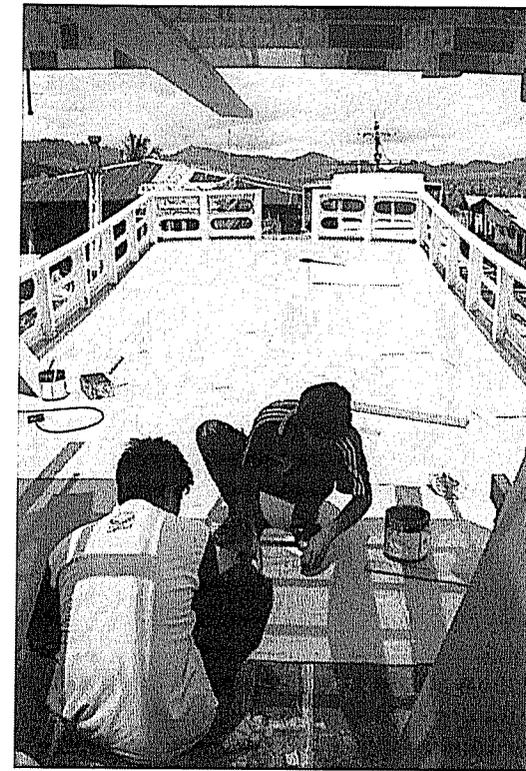
The new deck was not constructed in a traditional way and with traditional material, but with plywood, glass fibre mats, and polyester to make it more durable.
